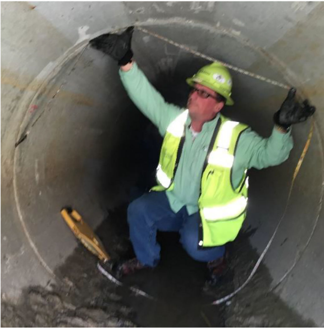
FIG. 1 Person Entry Inspection
